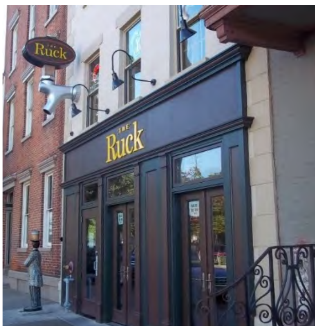
The completed project restored a pub type façade and corrected the poor window choices above. Creative signage was also installed.
