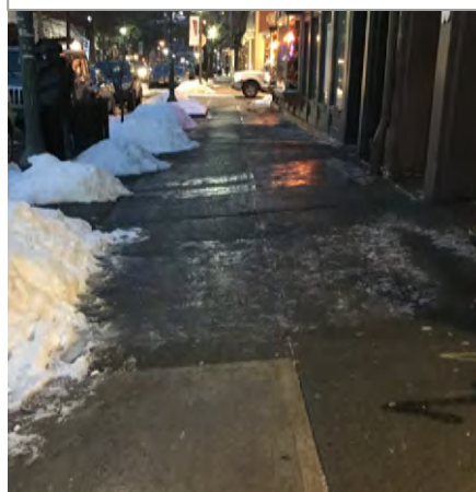
Don't allow building drainage to drip on a sidewalk and create dangerous icing.
