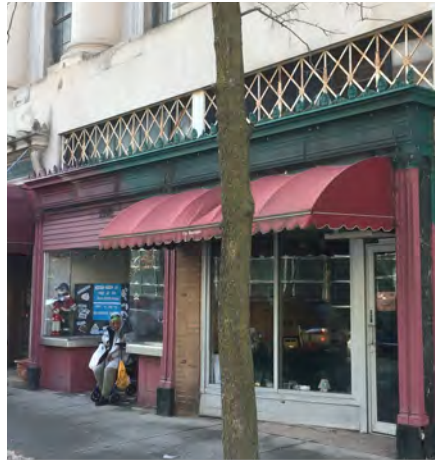
Modern aluminum storefronts are not allowed and two storefronts in the same building should match each other.
