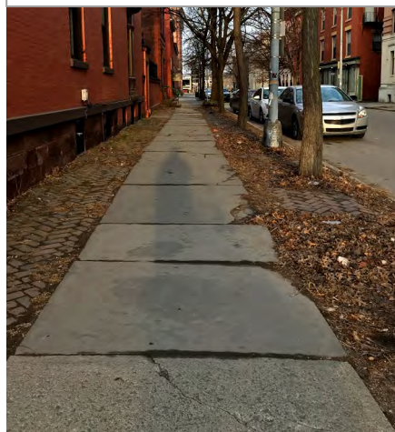
Slate/Bluestone can be reset by an experienced mason. It has lasted 100 years and can serve many more decades.
