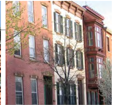
Some brick needs to be painted, some does not.
