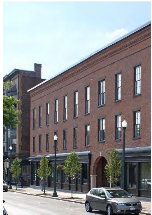
The Chazan Building renovation restored an arched entry on Broadway that had been hidden by earlier inappropriate work.
