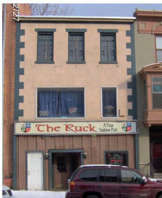
An inappropriate 1970’s renovation interrupted the window rhythm and fortified the traditional storefront.
